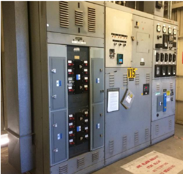
Figure 1 Final installation showing all seven (7) IR windows installed
