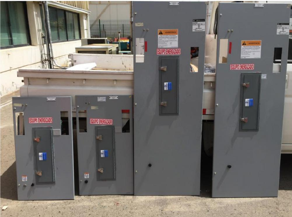
Windows installed on Equipment Doors before remounting to the Switchgear
