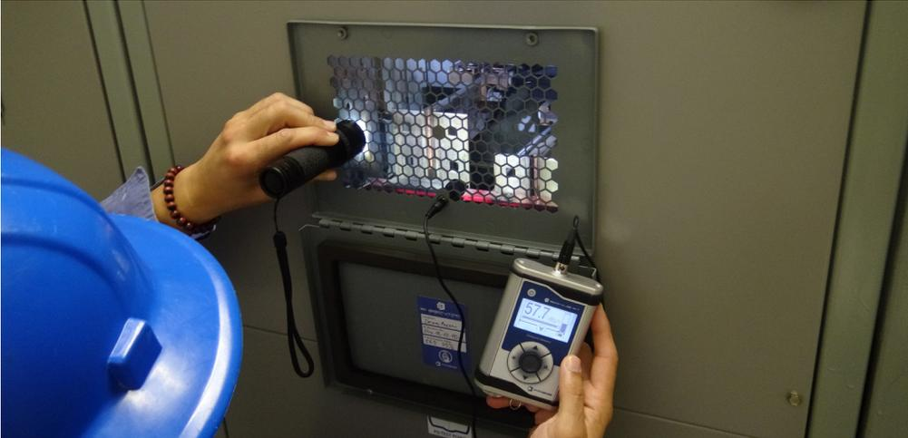
Custom sized windows were chosen to reduce the total installation cost and ensure that a single window would be sufficiently sized to see all the possible targets of interest in the equipment.
