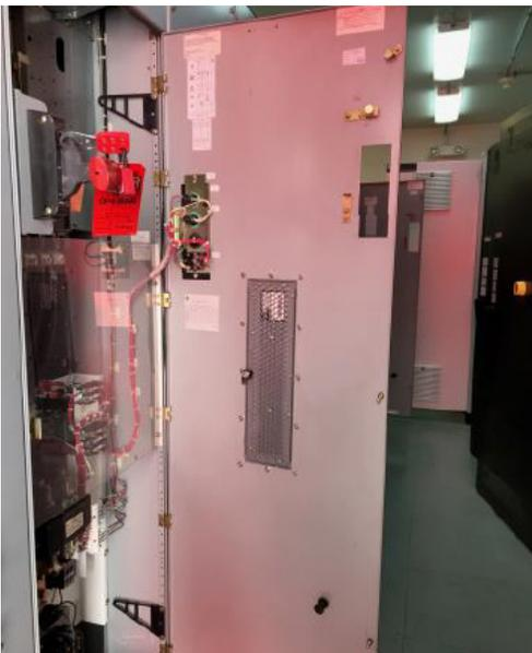
Switchgear door remounted with custom 20"x7" CAP-CT window fitted
