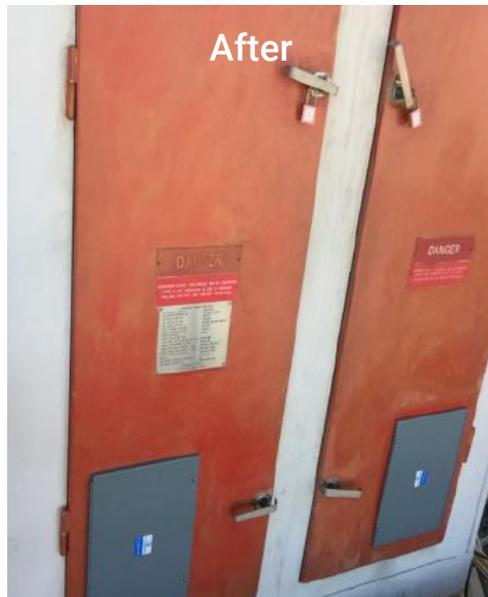
20"x16" CAP-ENV Windows installed on Generator Panels
