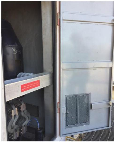
Windows were installed on lower portion of doors to give viewing of Incoming Connections
